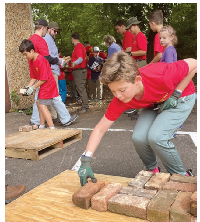
A Scout uses a modified herringbone pattern, the ultimate interlocking technique for heavy, irregular building materials.
