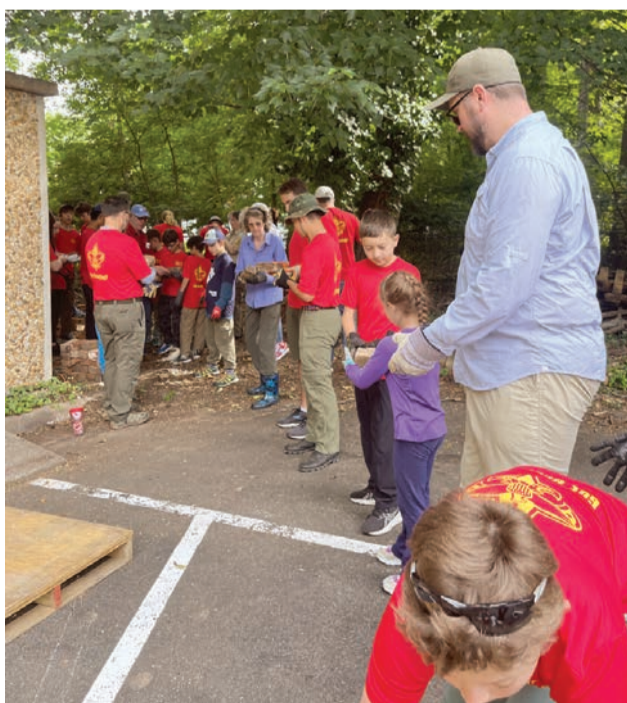
The Scouts form a "bucket brigade" to pass the bricks from one person to another to move them from behind the dumpster to pallets that will be moved to Town of Vienna property.
